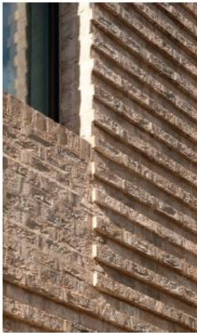
PROJECTING BRICK DETAIL - 15MM
